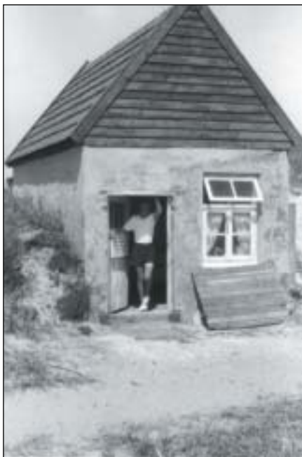
Station Wangerooge Ost 1952
